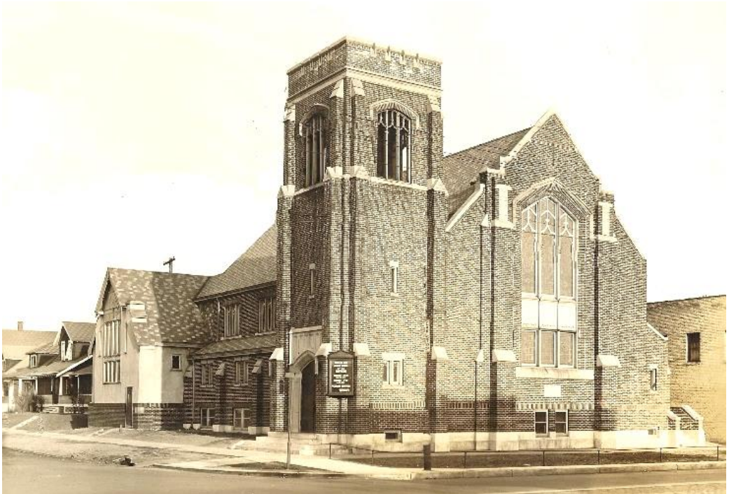
The church structure built in 1928. See also the first 1924 church on the left, which was attached behind and was used for classes.
